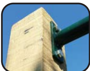
Drill and fix coach screws
